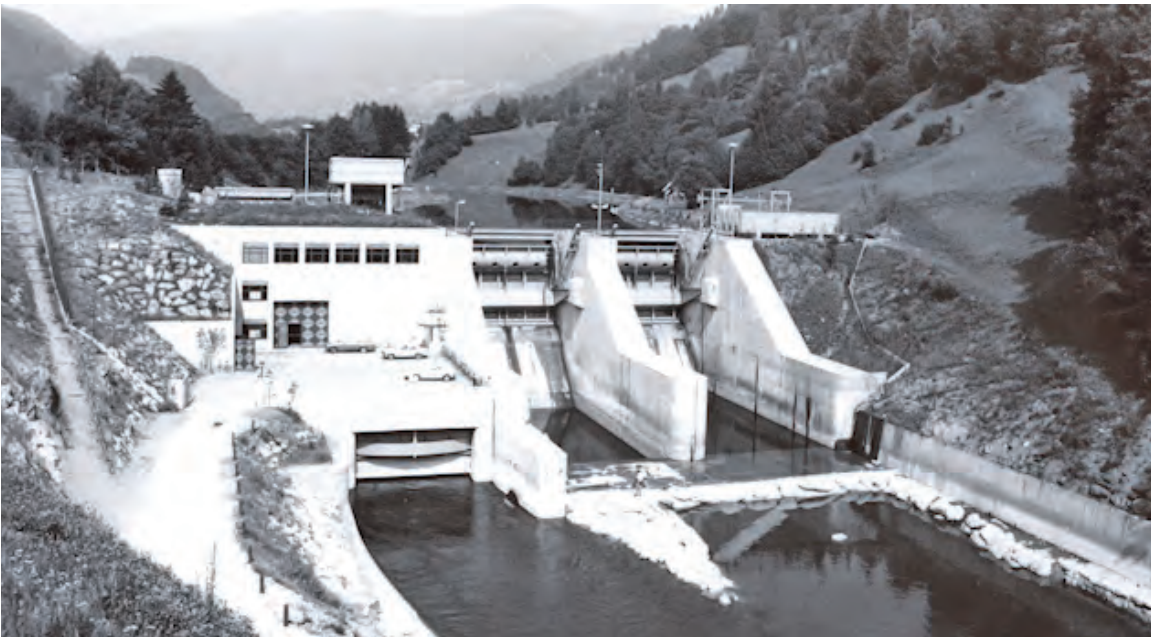
■ Hydro power station St. Georgen [VERBUND]
